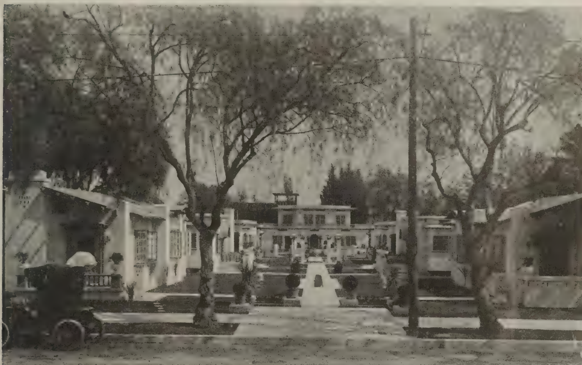
A BUNGALOW COURT, PASADENA, CAL., SHOWING SIX SINGLE HOUSES AND ONE DOUBLE HOUSE.
